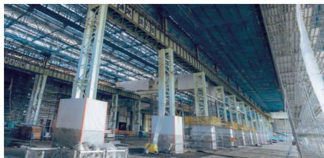
A look inside the press facility during renovations
